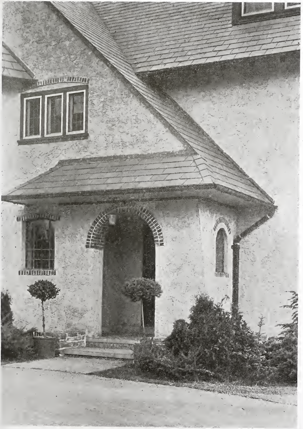
ENTRANCE DETAIL—RESIDENCE OF H. W. SELLERS. Horace Wells Sellers, Architect.
